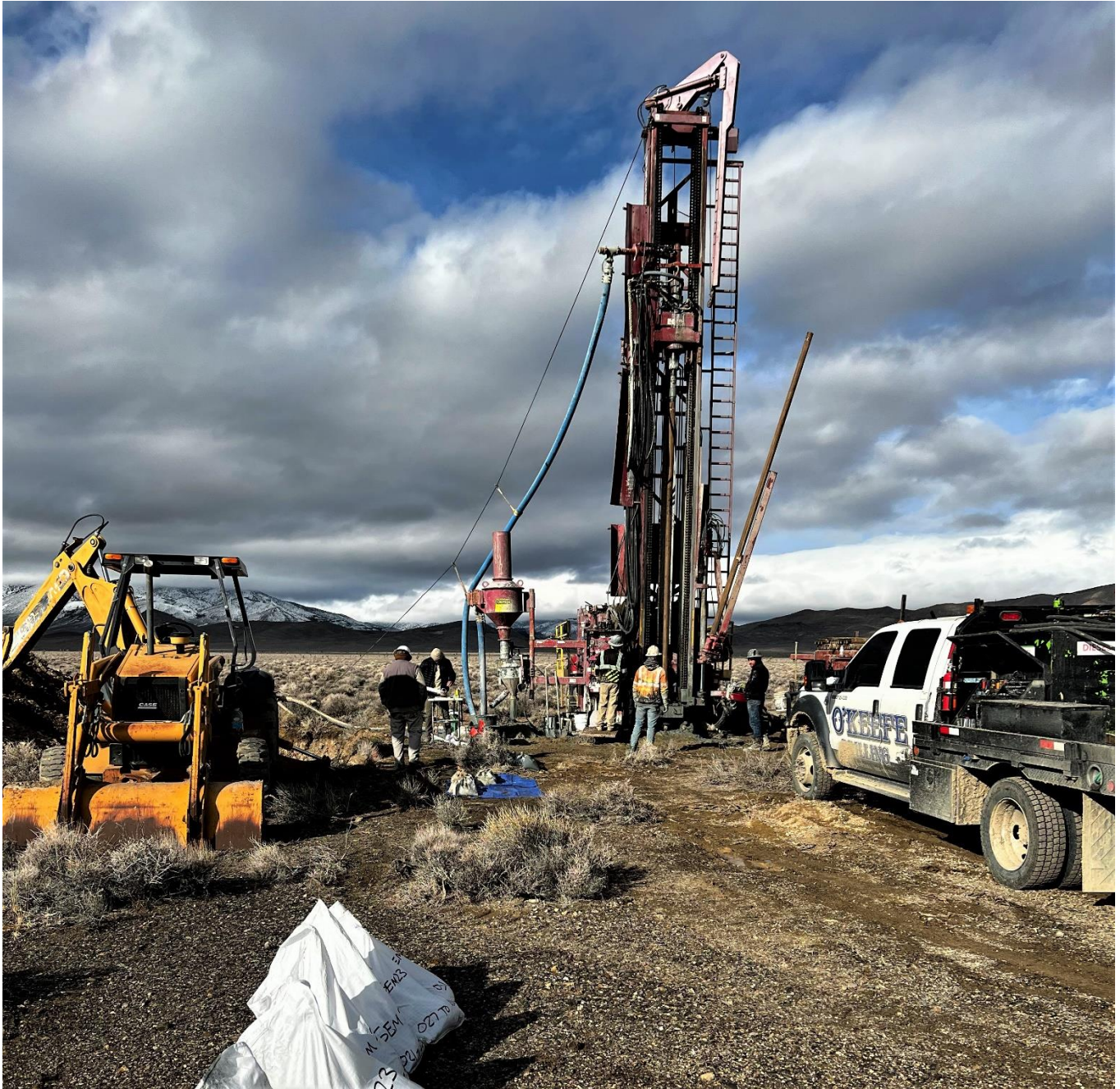
GEM23-04 Drilling in Progress, January 2023
